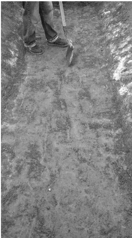
Fill above the barrel vault.
