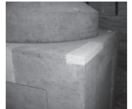
is removed and the edges of the cut-out are honed smooth. Straight line seams between old and new stone may give way under pressure in the future, so the cut-out and inserts are carved into other-than-right angled shapes to protect the seam.
